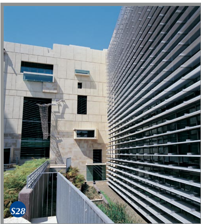
Neville Bonner Building, Brisbane, Qld. – SS203/60 louvre tiered panels supported by structural “T” section frame.
